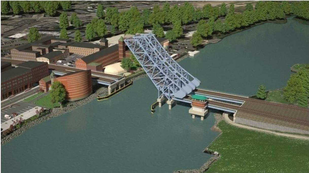
Figure ES-3—Rendering of Bascule Bridge in the Open Position (Option 4S)
