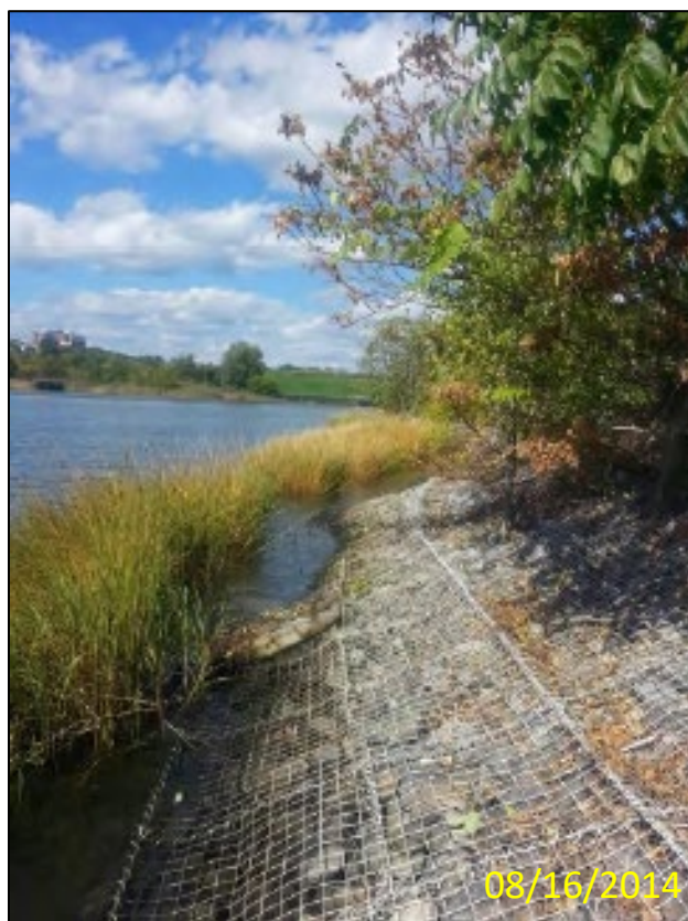
Photo 14 – Gabion slope along Norwalk River (looking north).
