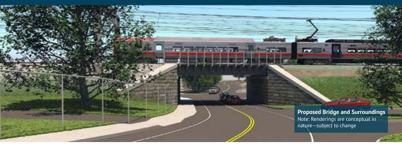
The New Haven Line passing through Norwalk relies on infrastructure from the 19th century. To modernize, this project replaces the Fort Point Street bridge and the neighboring walls supporting the track. The project realigns Fort Point Street with S. Smith Street, increasing safety and improving visibility for drivers and pedestrians.
