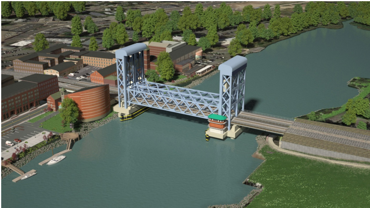
Figure ES-8—Rendering of the Long Span Vertical Lift Bridge in the Closed Position (Option 11C)
