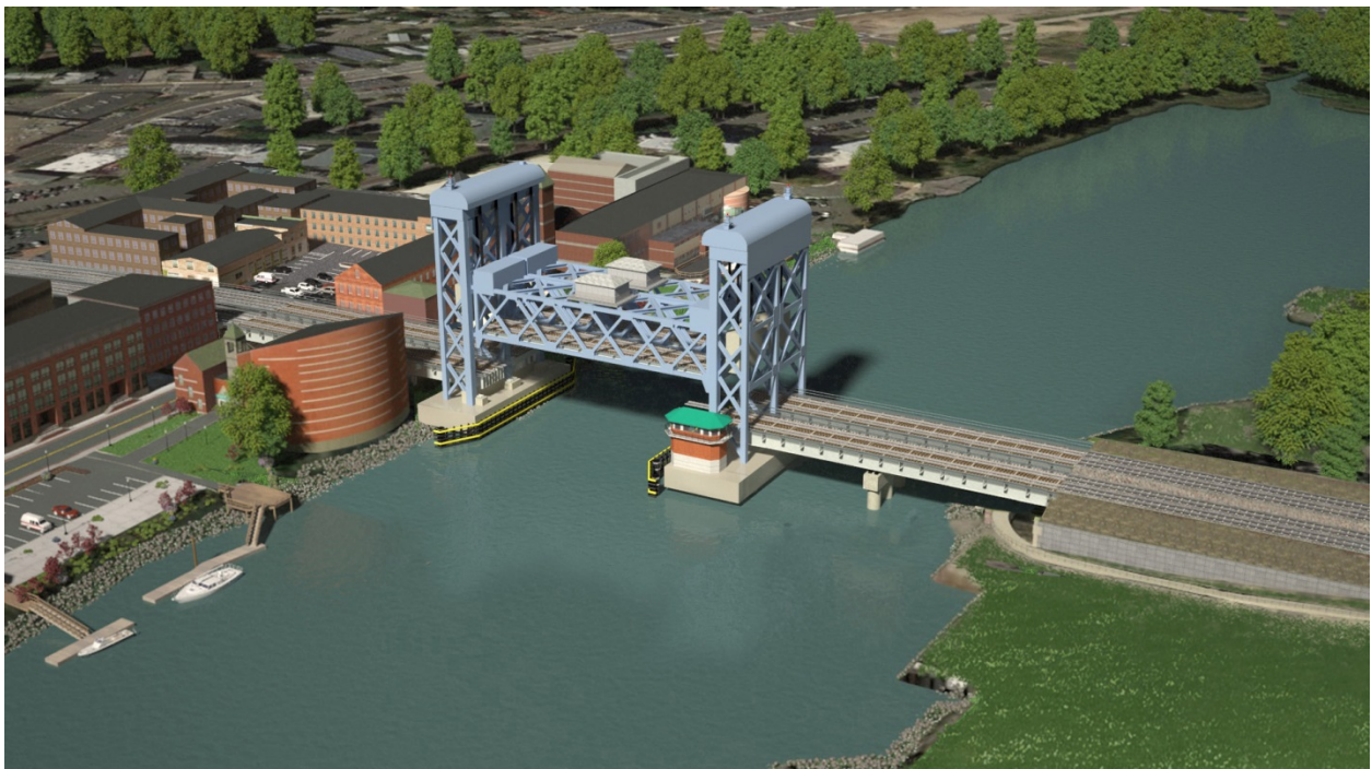
Figure ES-6—Rendering of the Short Span Vertical Lift Bridge in the Open Position (Option 8A)
