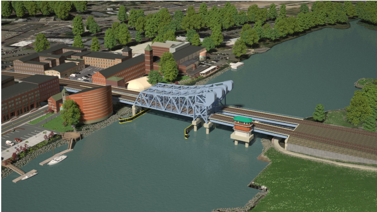
Figure 2-3—Rendering of Bascule Bridge in the Closed Position (Option 4S)
