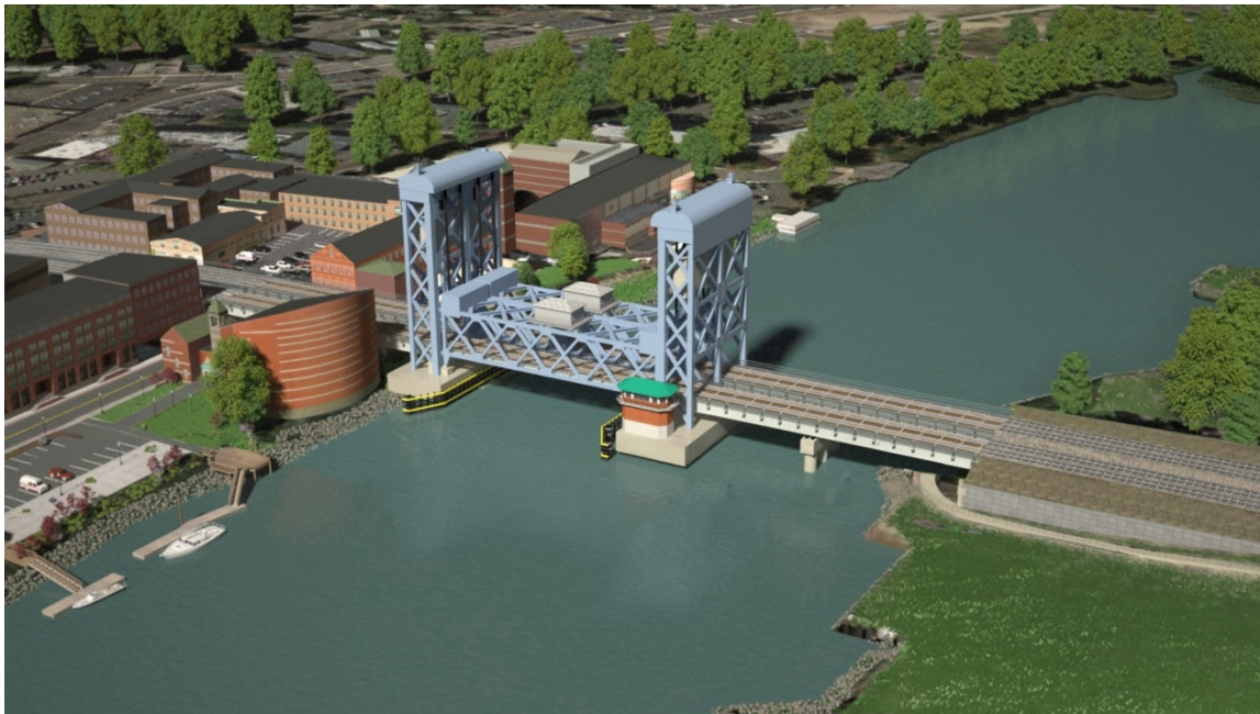
Figure 2-7—Rendering of the Short Span Vertical Lift Bridge in the Closed Position (Option 8A)
