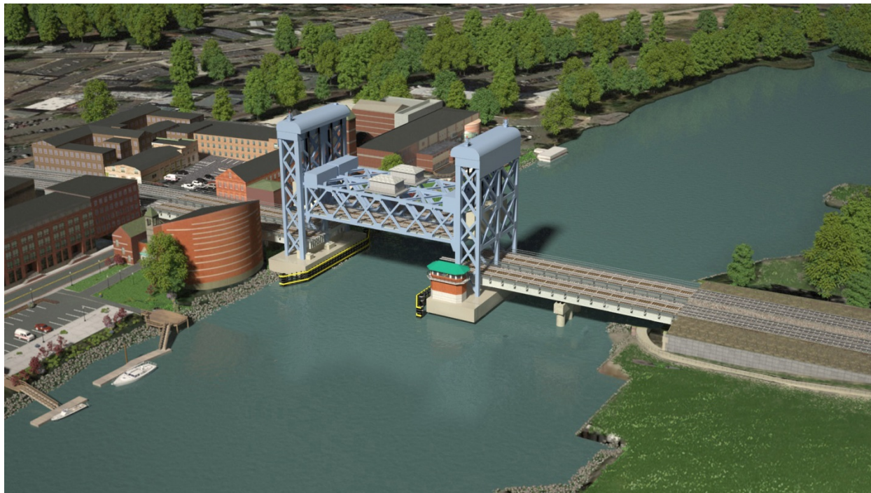
Figure 2-8—Rendering of the Short Span Vertical Lift Bridge in the Open Position (Option 8A)
