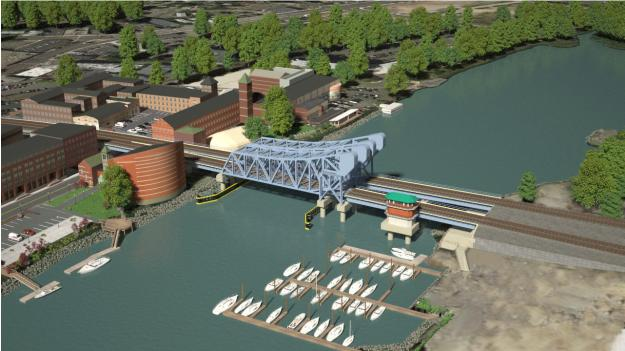
Figure ES-2—Rendering of Bascule Bridge in the Closed Position (Option 4S)
