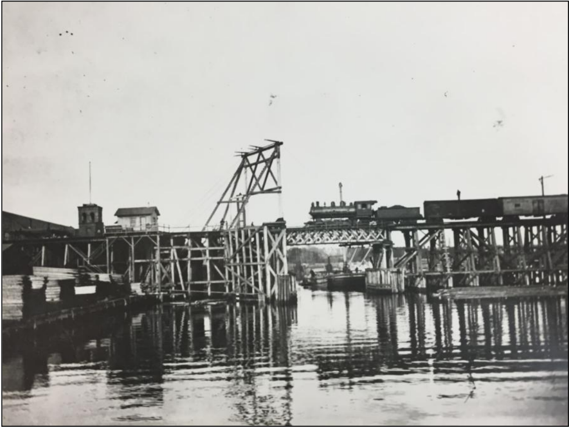
Image 8. Train going over the tracks on the Norwalk Walk Bridge ca. 1913 (construction of the new Washington Street Bridge is in the foreground) (Norwalk History Room, Norwalk Public Library).
