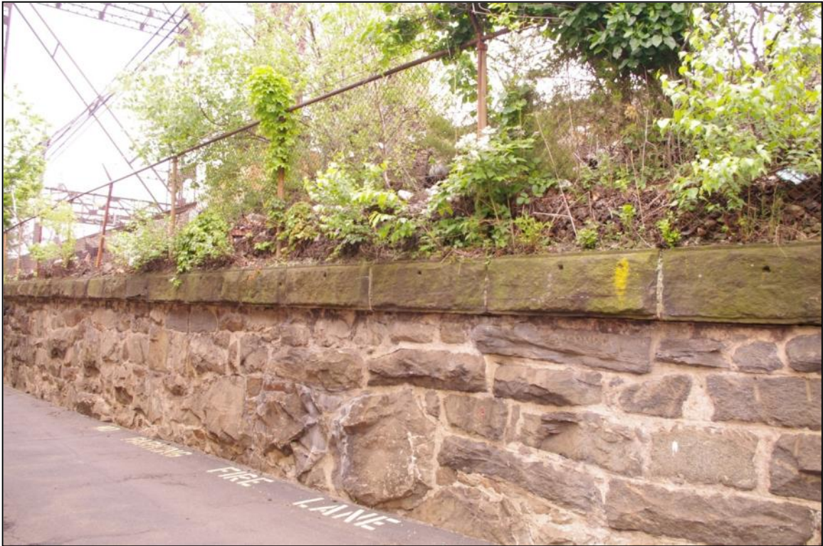
Photograph 7. Typical section of stone retaining wall for the 1896 four-tracking and grade-separation project.
