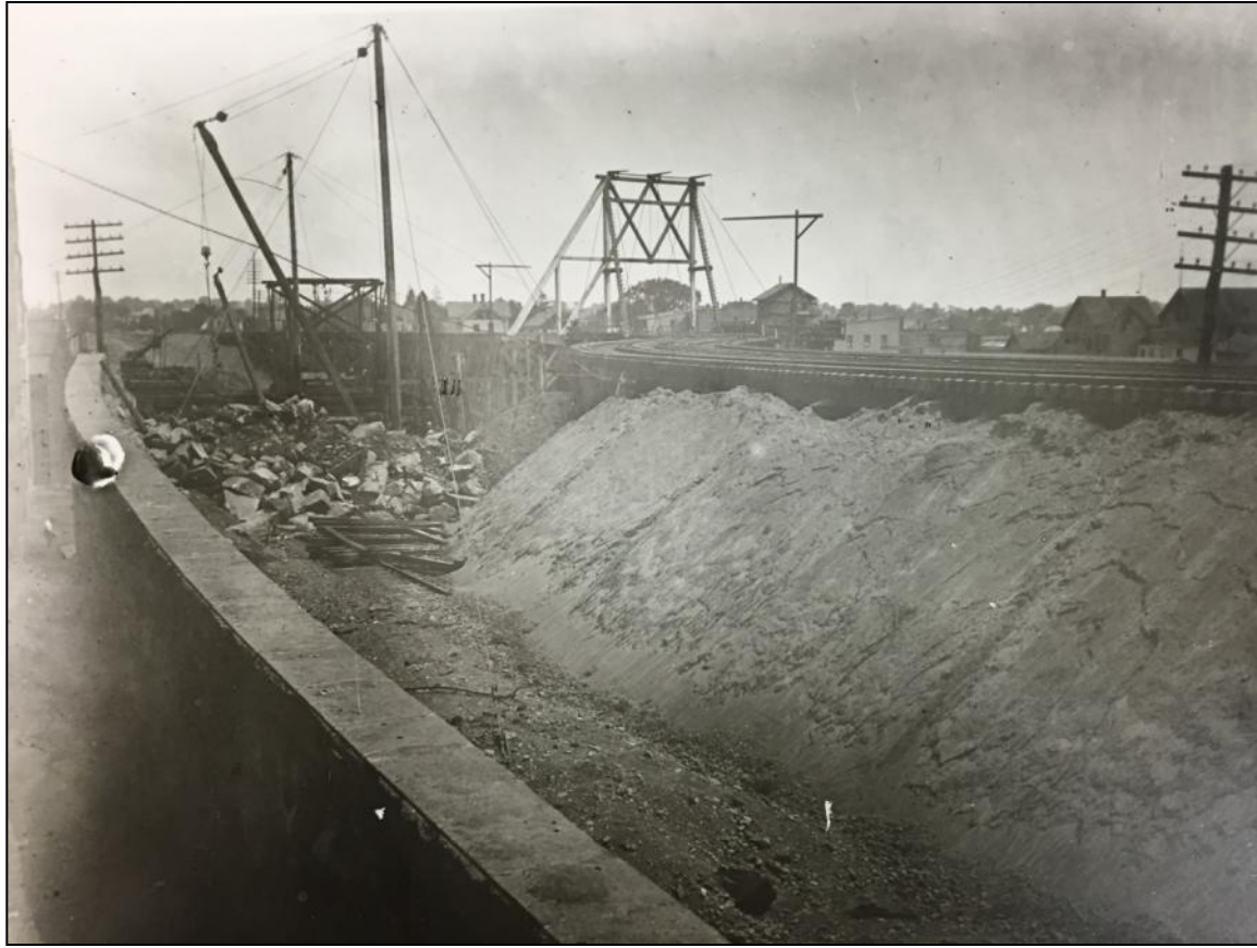
Image 3. View of massive retaining walls constructed to elevate the NY, NH & H line ca. 1895 (Norwalk History Room, Norwalk Public Library).
