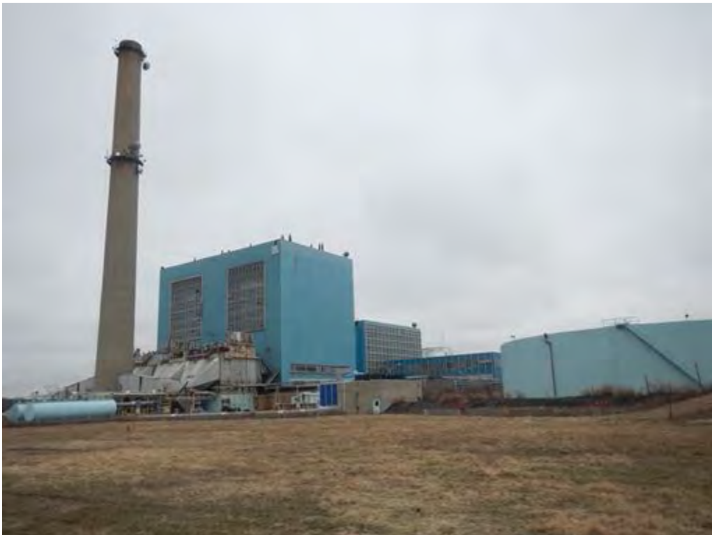
Photograph 12: View from Parcel 5/86/1, looking northwest within the Staging and Storage Area at the power plant. Facing northwest. 3/12/2020.
