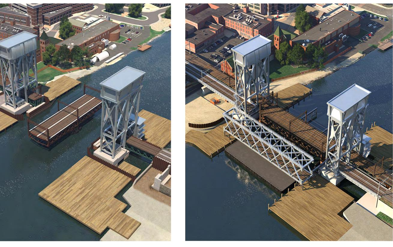
The Vertical Lift Bridge design allows the existing swing span to remain operable during approach, pier and tower construction. The lift span will be built off site and brought in by barge.
