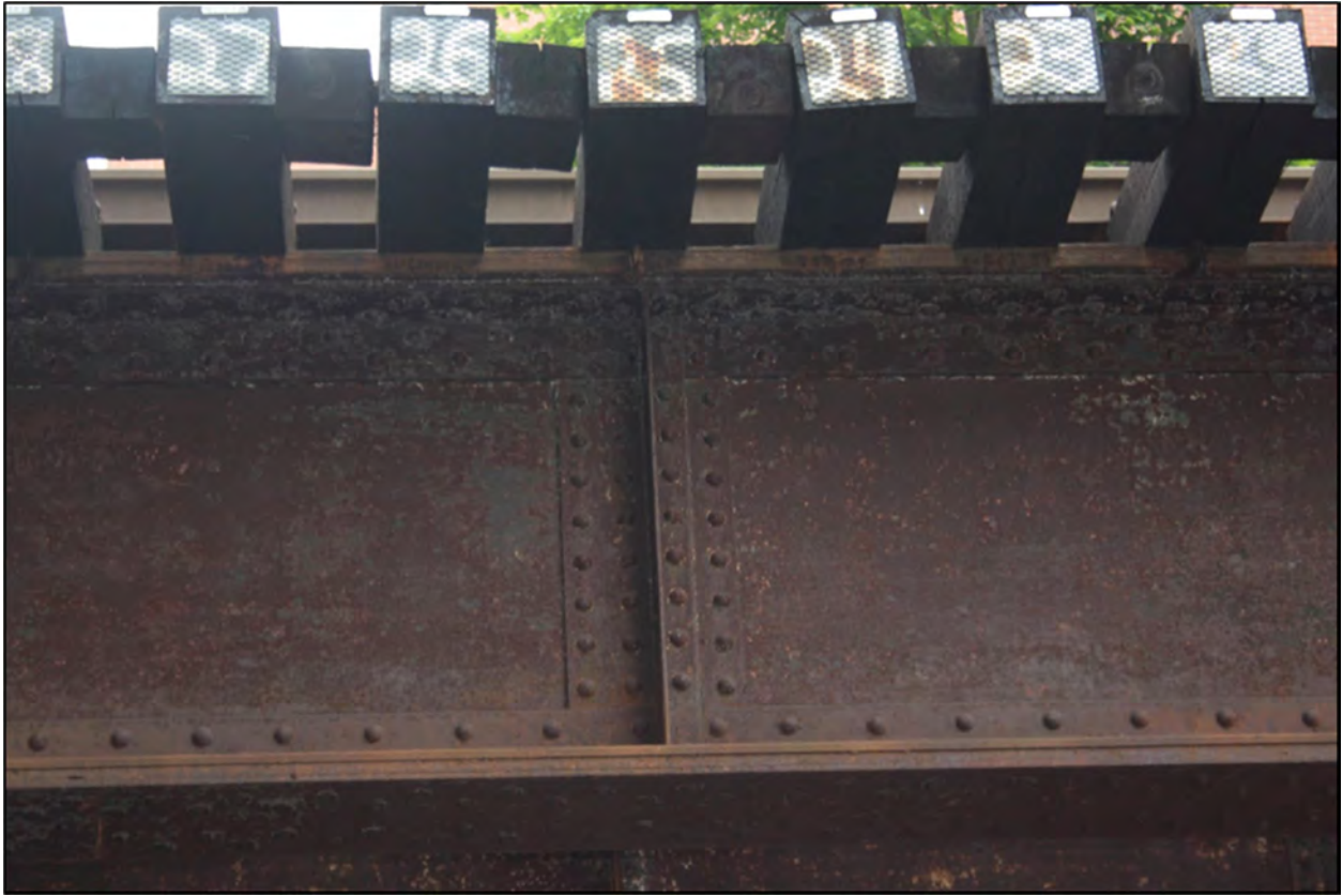
Photograph 28: Ann Street Bridge, detail of stiffener and bottom flange, camera facing east.
