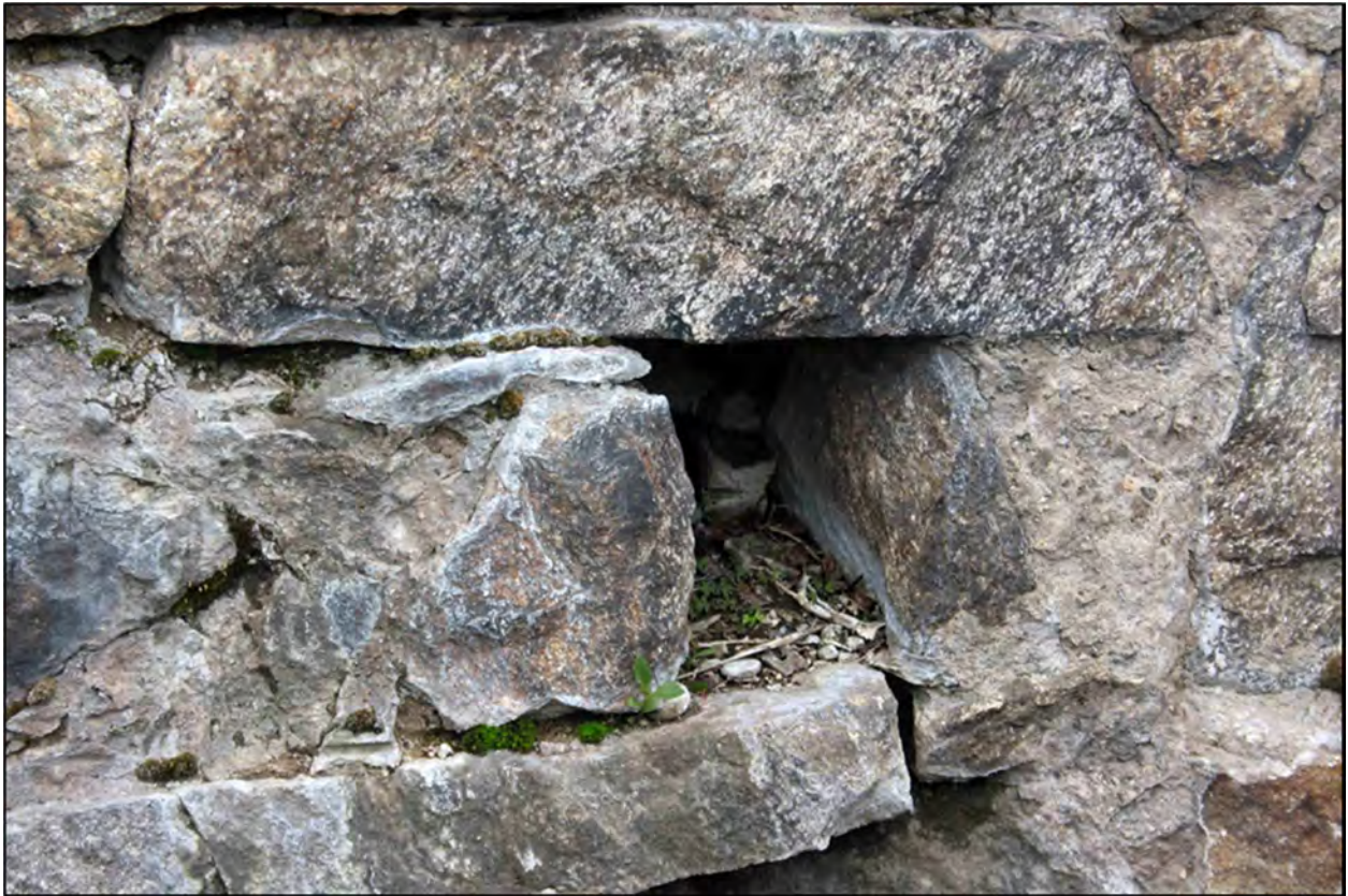
Photograph 36: Retaining wall south of Marshall Street, detail of weep hole, camera facing east.
