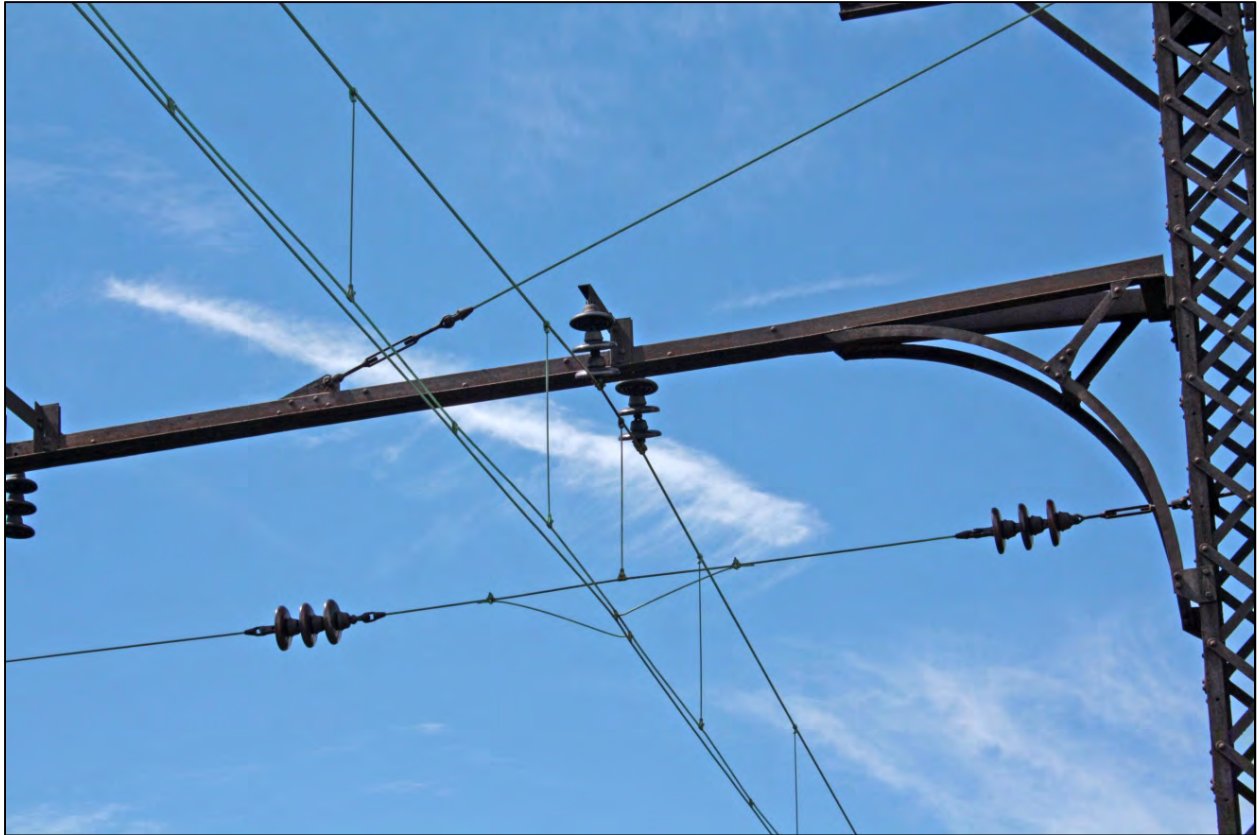
Photograph 13: Detail of overhead strut and catenary connection, braced H-column and lattice-pole type, camera facing south.
