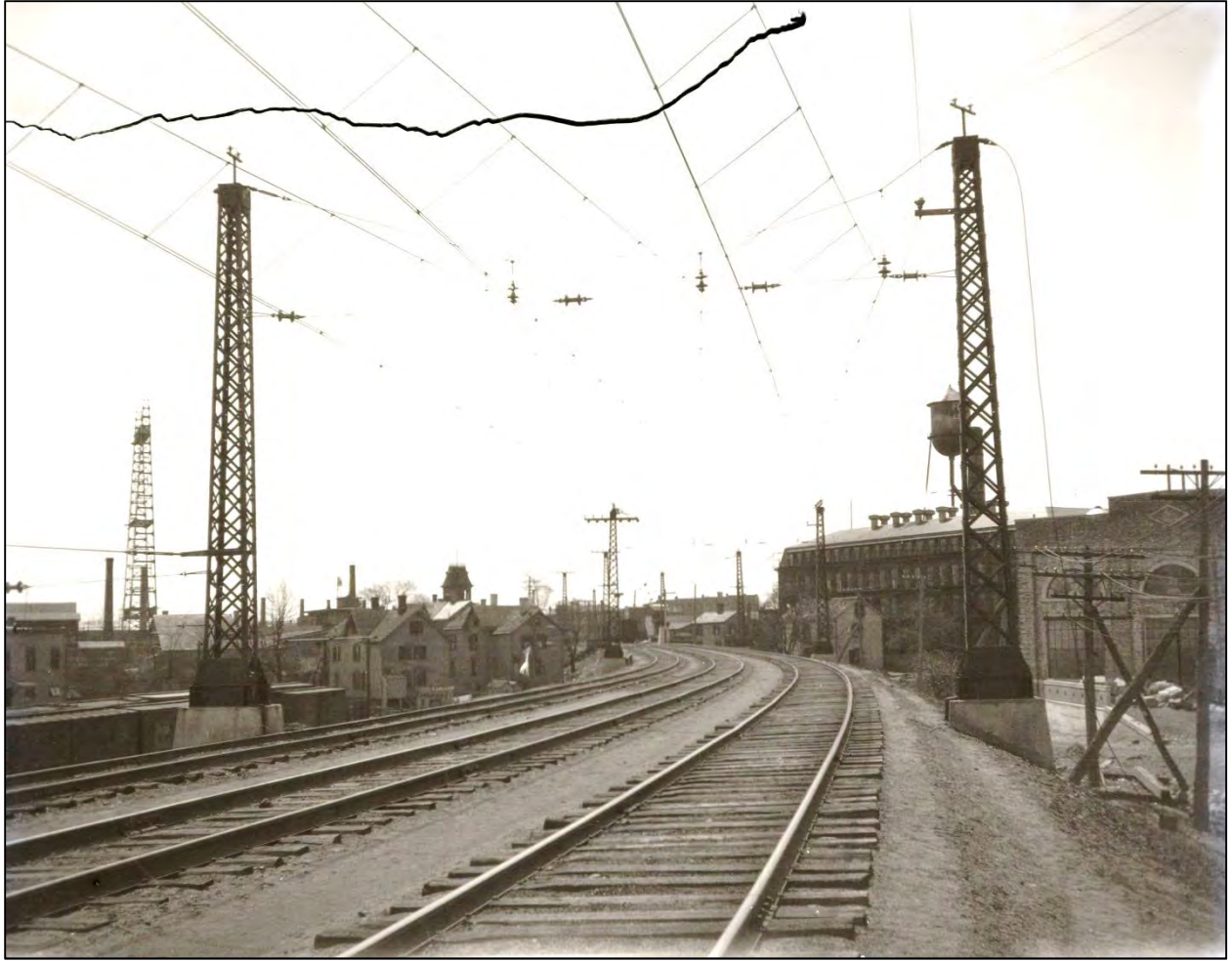
Figure 8: Dock Yard catenary, Harry F. Brown photograph, April 1914, looking south, with the tower of the Norwalk Lock building visible in the distance.
