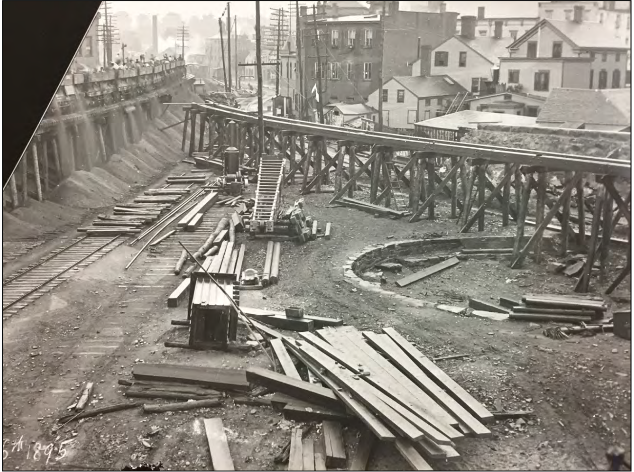
Figure 4: Beginning of construction to elevate the Danbury branch as part of the raising of the main line, 1895 (Norwalk History Room, Norwalk Public Library). Wooden trestles support a single track, over which dump cars with fill will travel to create a raised embankment; the dump cars for the main line are visible in operation at the left. The buildings are the backs of the ones along the east side of North Main Street. The stone circle is the remnant of the small turntable shown in Figure 3.
