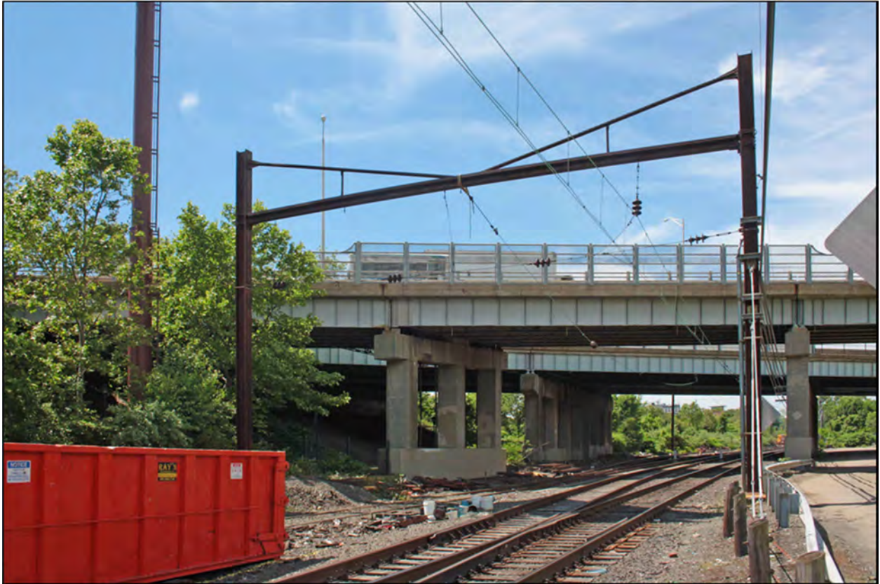
Photograph 15: H-column-type catenary support, ca. 1958, north of I-95, camera facing southwest.
