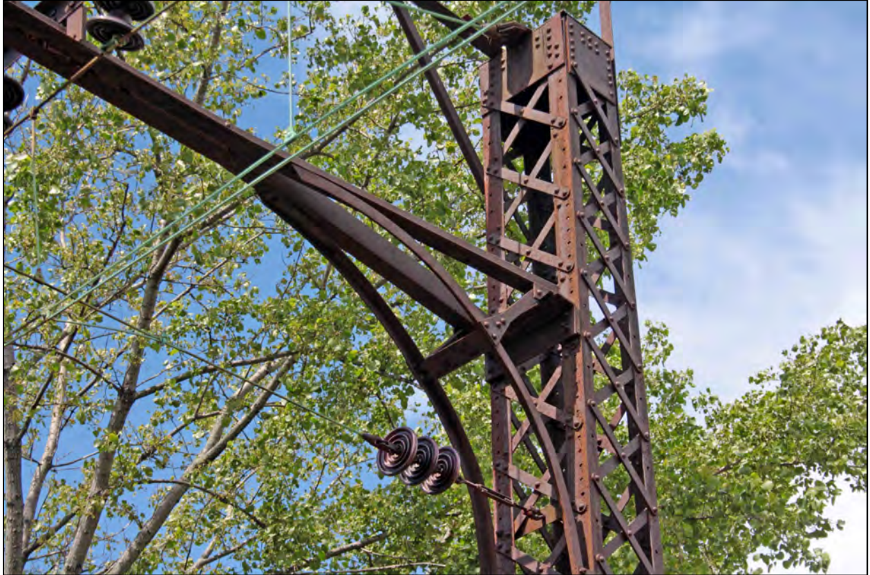
Photograph 12: Detail of brace, braced H-column and lattice-pole type, camera facing southwest.
