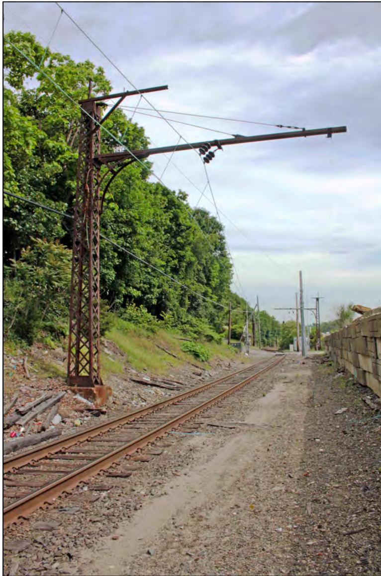
Photograph 3: Typical catenary support of the single lattice pole-bracket type used above single-track portions of the line, camera facing northeast.
