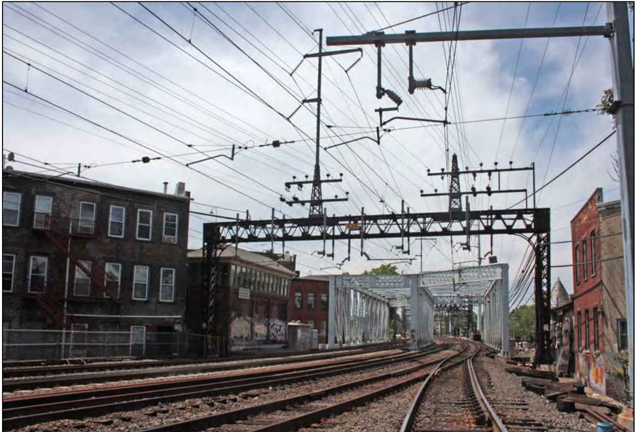
Photograph 1: Catenary Bridge 526, at the junction of the main line and Danbury line, camera facing southwest. This catenary structure is shared by the main line and Danbury branch.
