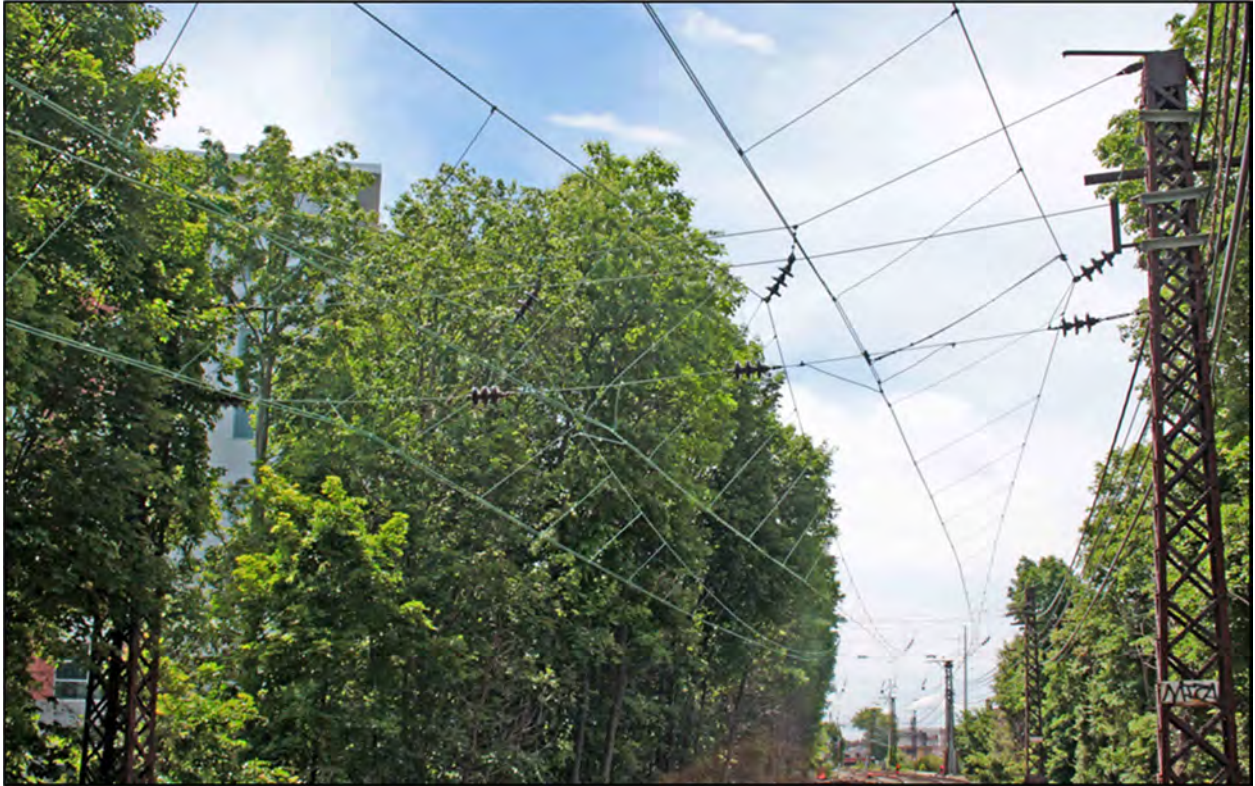
Photograph 10: Detail of three-track catenary, paired lattice-pole type, curved section, camera facing south.
