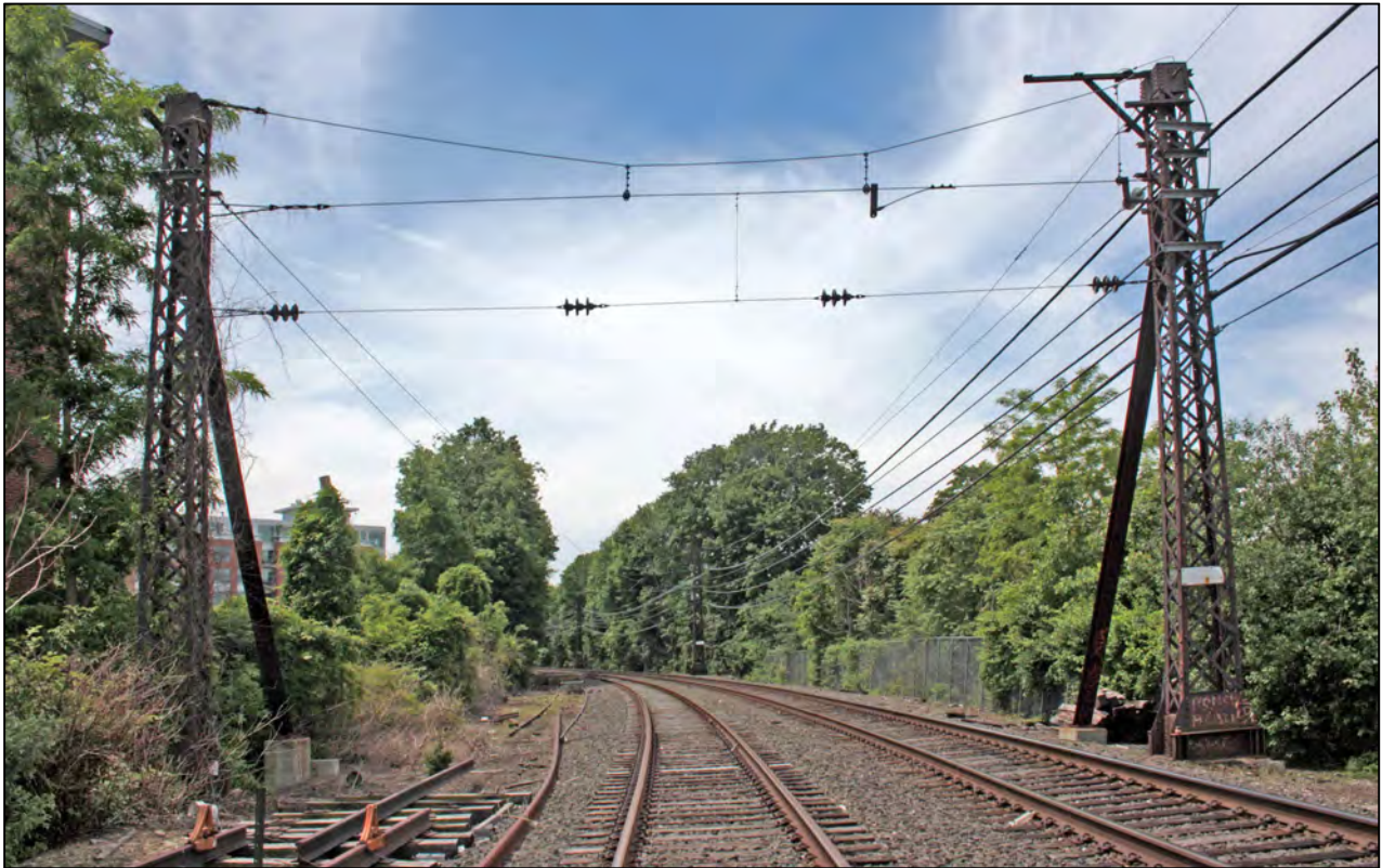
Photograph 7: Paired lattice-pole type, used for multiple-track situations, camera facing southwest. The bracing on the south sides of the poles is an alteration.
