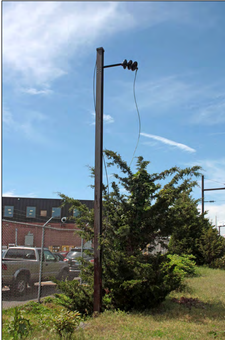
Photograph 16: Single H-column pole, probably intended for a guy wire, camera facing south.
