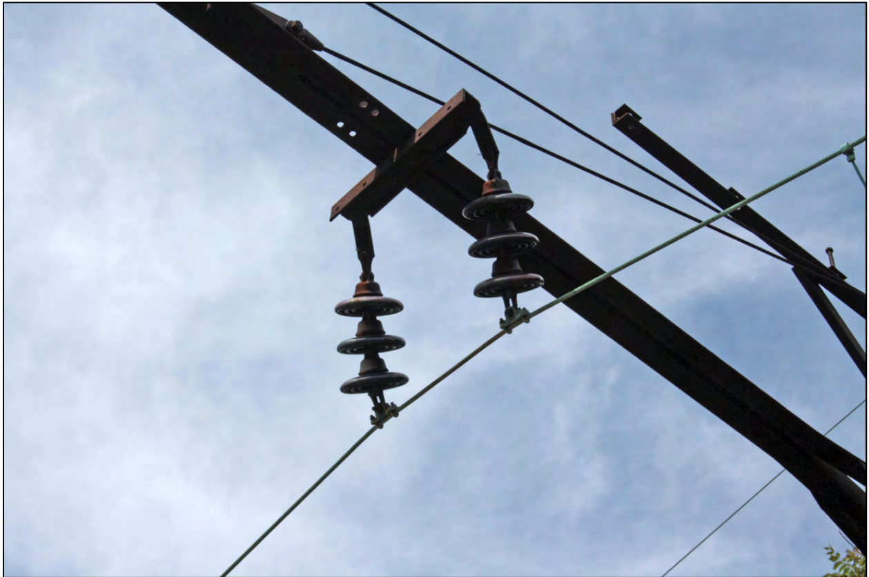
Photograph 4: Detail of insulators and catenary attachment, single lattice pole-bracket type, camera facing southwest.
