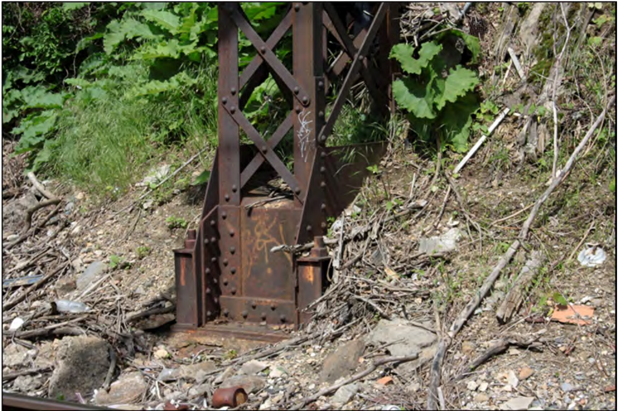
Photograph 5: Detail of footing, single lattice pole-bracket type, camera facing southwest.
