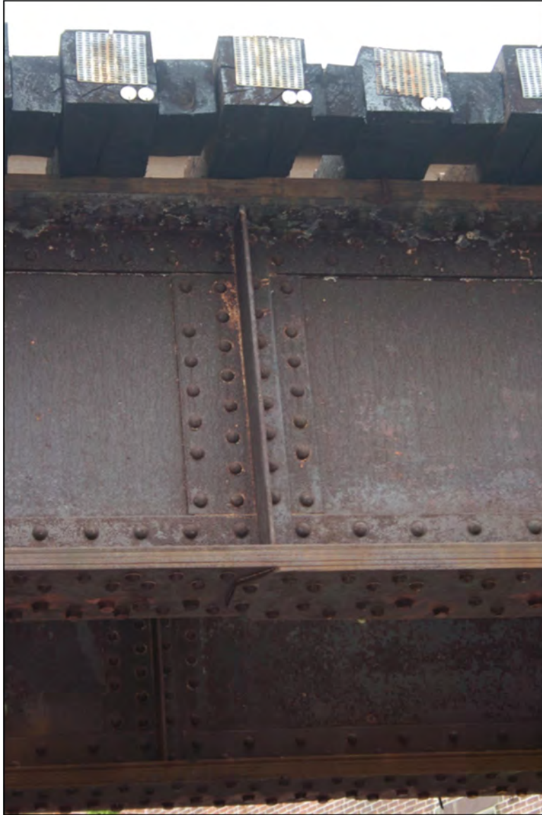
Photograph 21: Marshall Street Bridge, detail of stiffener and bottom flange, west side, camera facing east.
