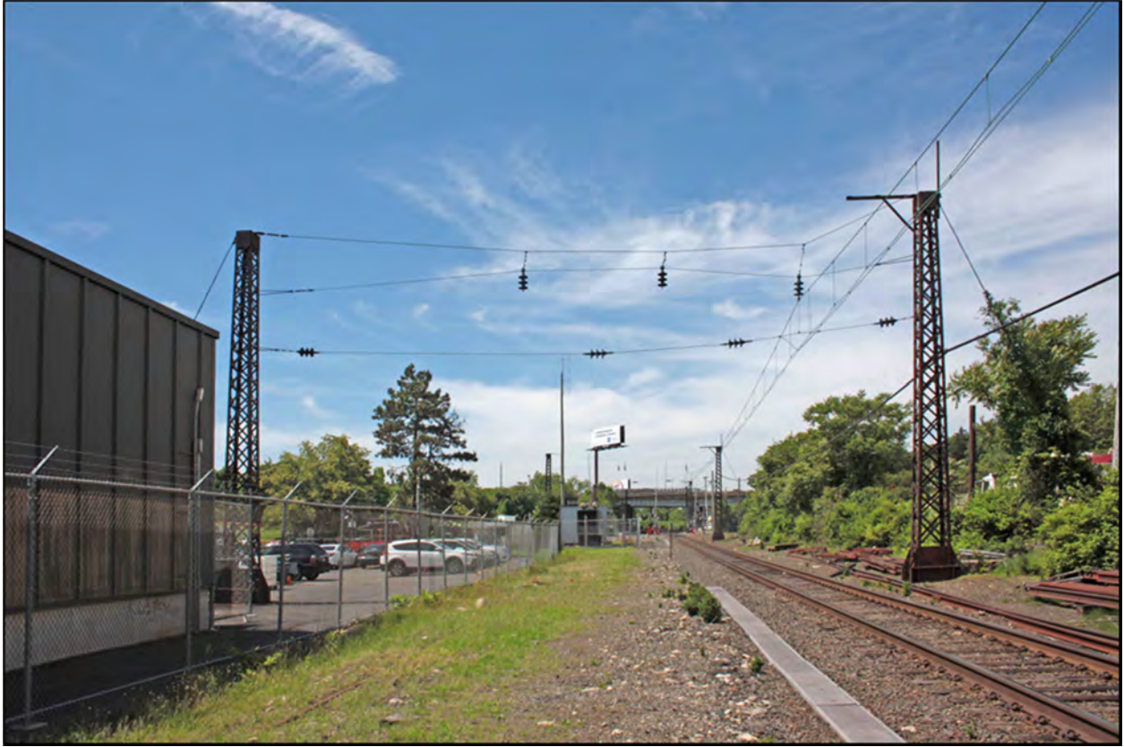
Photograph 6: Paired lattice-pole type, used for multiple-track situations, camera facing southwest.
