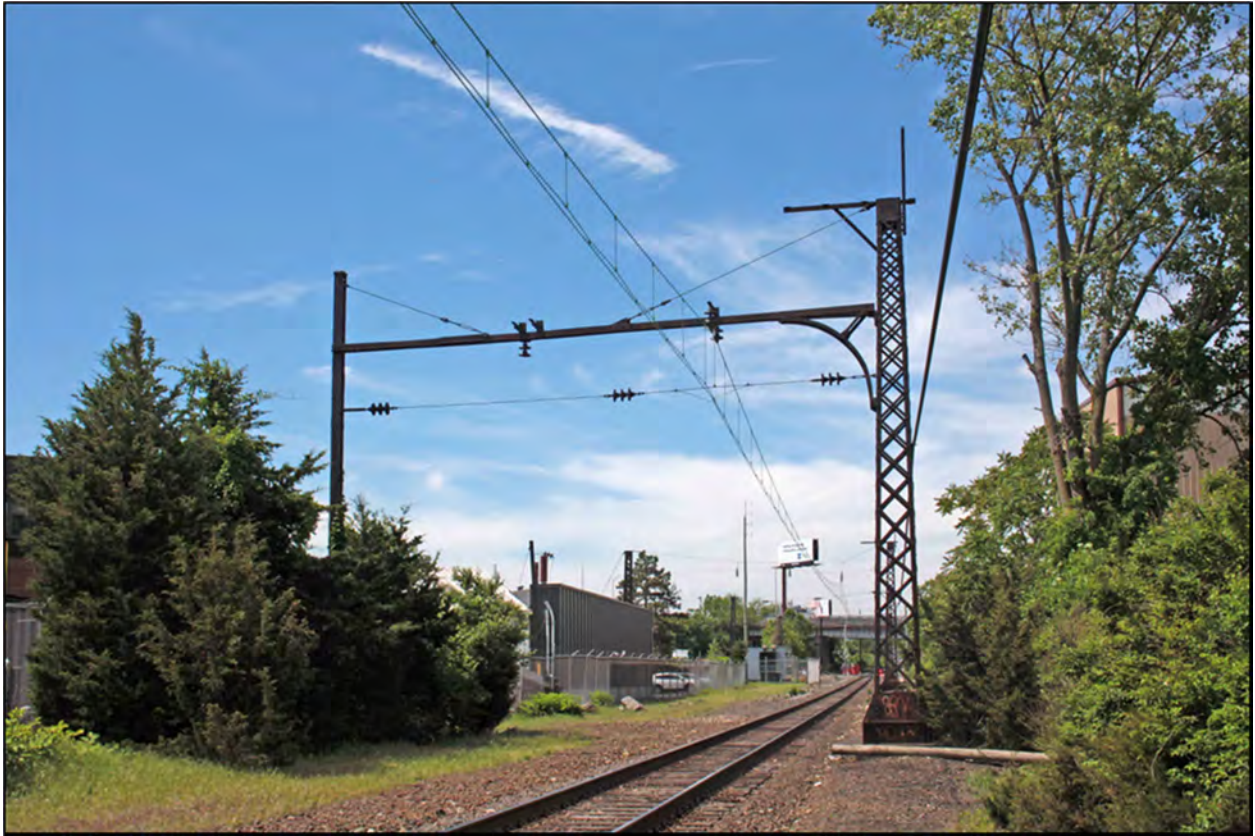
Photograph 11: Braced H-column and lattice-pole type, camera facing south.
