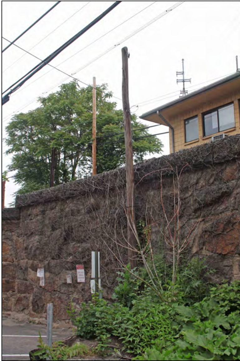
Photograph 35: Retaining wall south of Marshall Street, detail of clothesline pole attached to wall, camera facing northeast.
