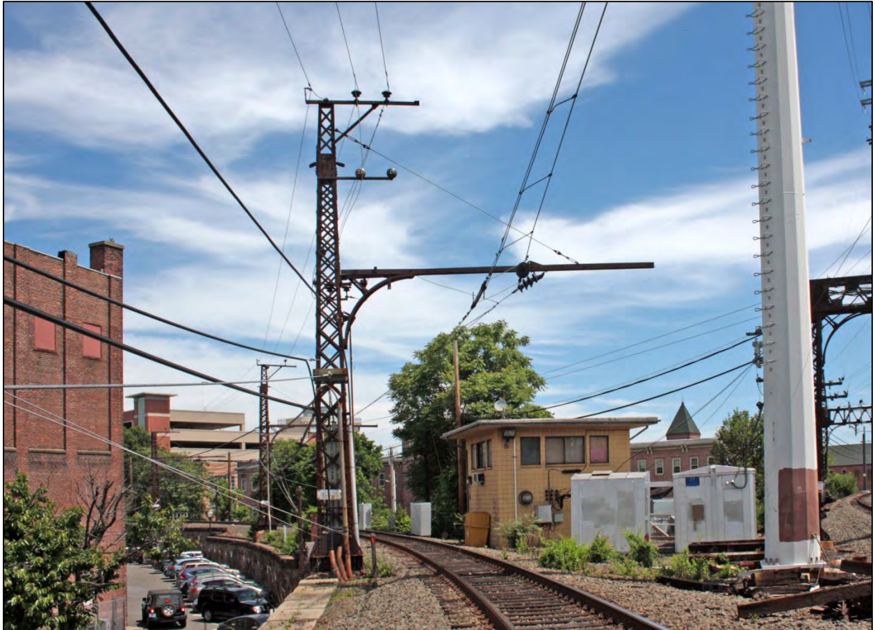
Photograph 2: Typical example of the single lattice pole-bracket type used above single-track portions of the line, camera facing northeast. The structure has a high extension to carry signal lines.
