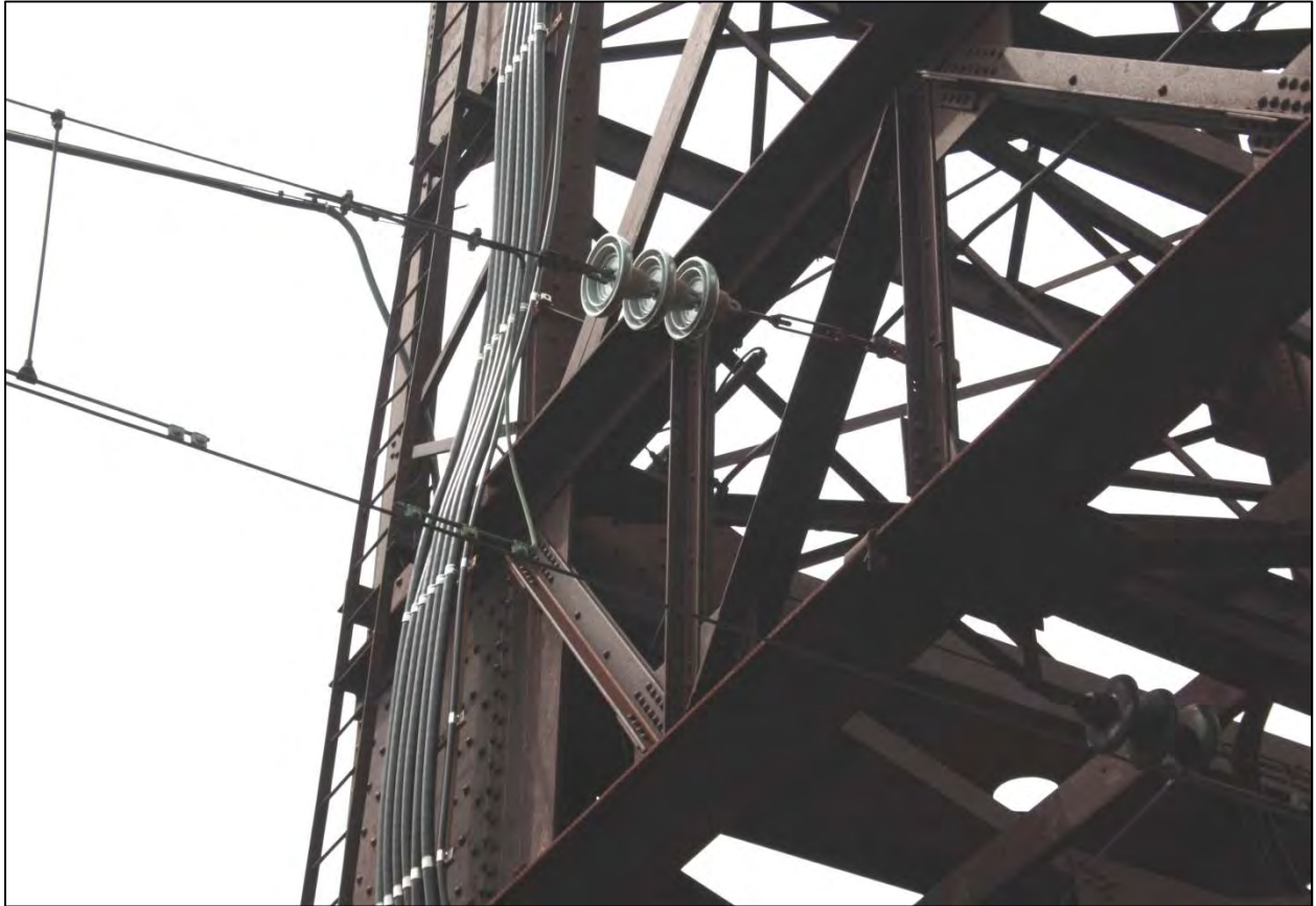
Photograph 22: West high tower (Bridge 577), Saugatuck River Railroad Bridge (Saga Bridge, Westport), detail of insulators and catenary wires, camera facing southwest.
