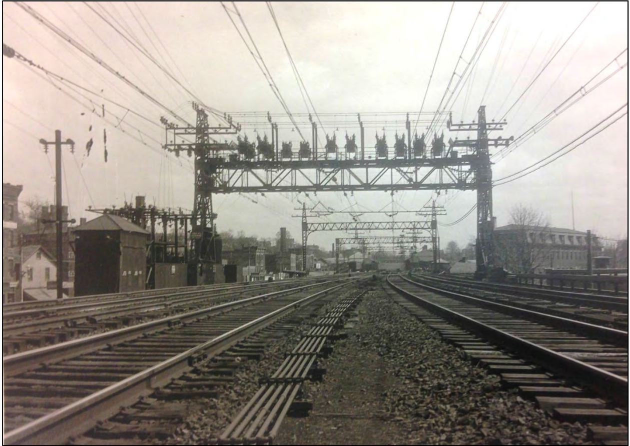
Figure 7: Anchor Bridge 524 (sectionalizing bridge) looking west, Harry F. Brown photograph, 1931.
