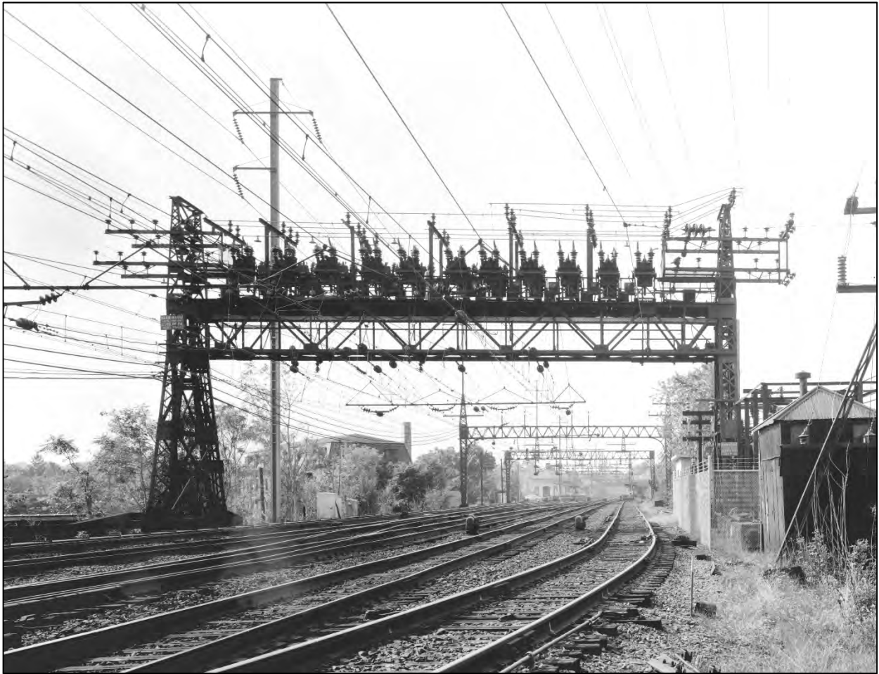
Figure 13: Anchor Bridge 524 (sectionalizing bridge) looking west, 1980, Historic American Engineering Record photograph by Thomas Brown, “New York, New Haven & Hartford Railroad, Automatic Signalization System (HAER No. CT-8).
