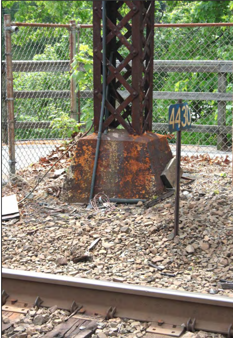
Photograph 26: Typical concrete footing for catenary supports (Bridge 578, south support, Westport), camera facing south.
