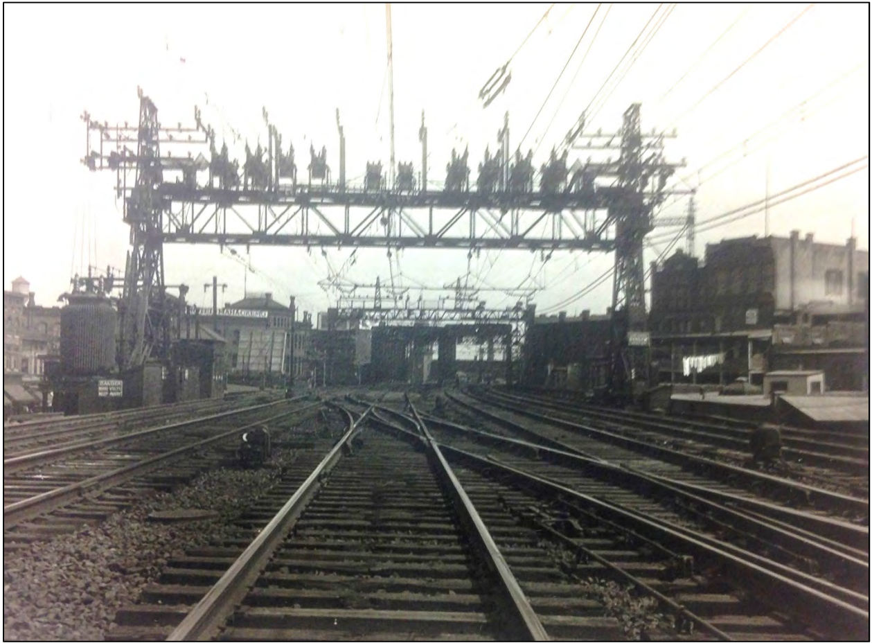
Figure 6: Anchor Bridge 524 (sectionalizing bridge) looking east, Harry F. Brown photograph, 1931.
