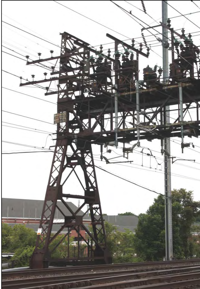
Photograph 3: Anchor bridge (sectionalizing bridge), Bridge 524, detail of south support, camera facing south.
