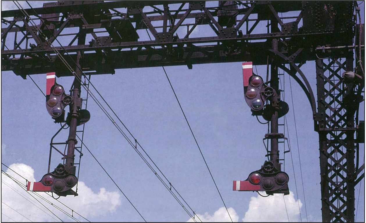
Figure 3: Lighted semaphore signals at the approach to the Saugatuck River Railroad Bridge. Undated photograph by T. J. Donahue (Lynch 2008). Many of the catenary structures along this portion of the line would have been fitted with similar signals.
