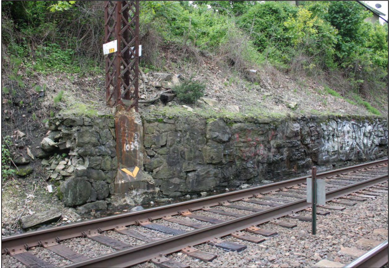
Photograph 13: Example of catenary pier built into low retaining wall, Bridge 553 (Norwalk), camera facing south.
