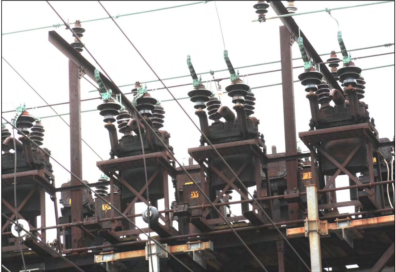
Photograph 4: Anchor bridge (sectionalizing bridge), Bridge 524, detail of electrical equipment mounted above tracks, camera facing southwest.
