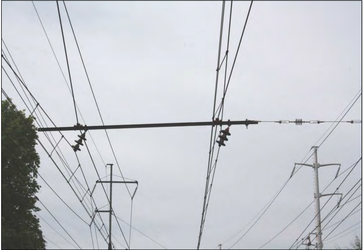
Photograph 14: Beam-type hangar, west of Westport Station, camera facing west.
