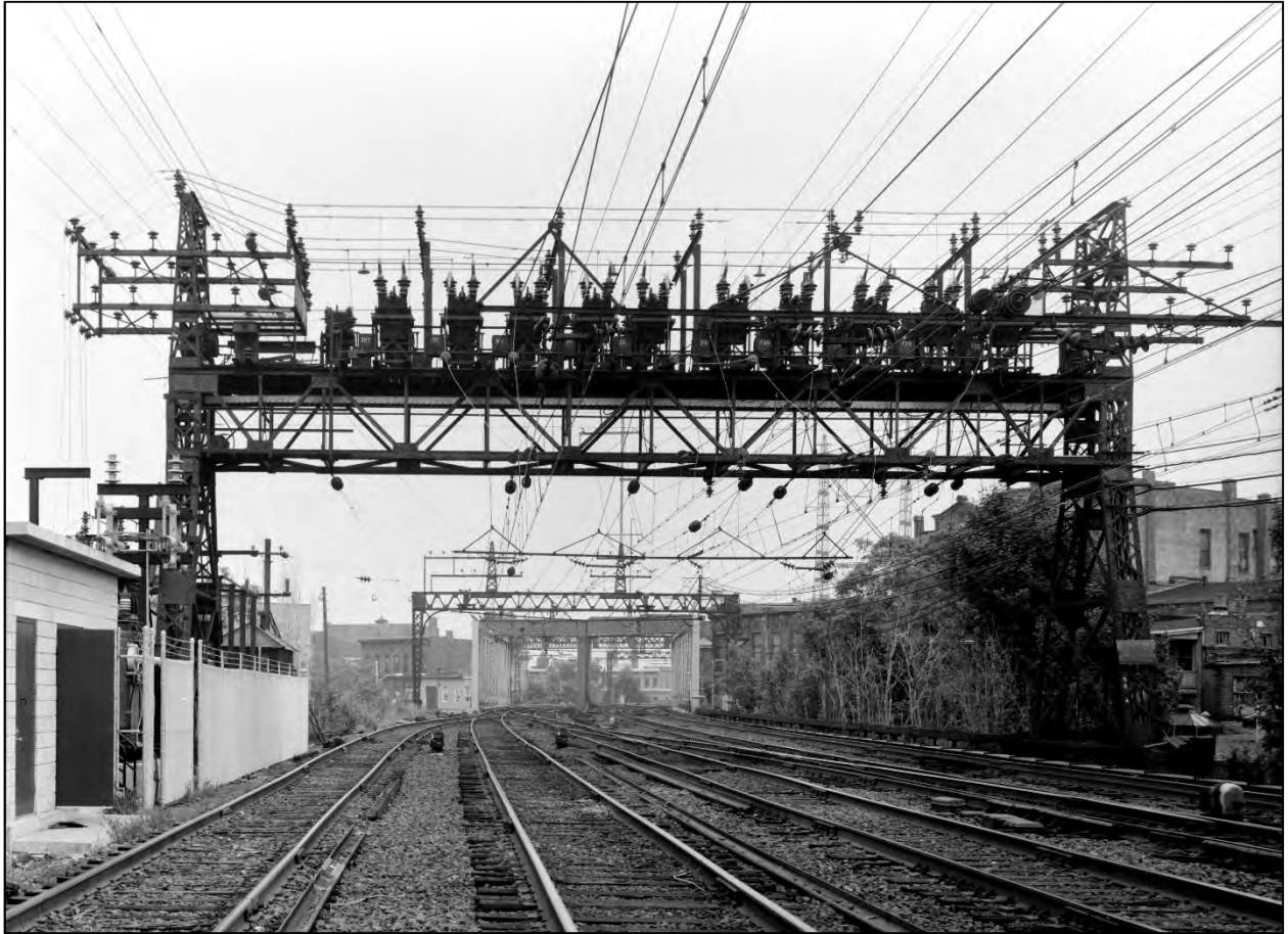
Figure 12: Anchor Bridge 524 (sectionalizing bridge) looking east, 1980, Historic American Engineering Record photograph by Thomas Brown, “New York, New Haven & Hartford Railroad, Automatic Signalization System (HAER No. CT-8).
