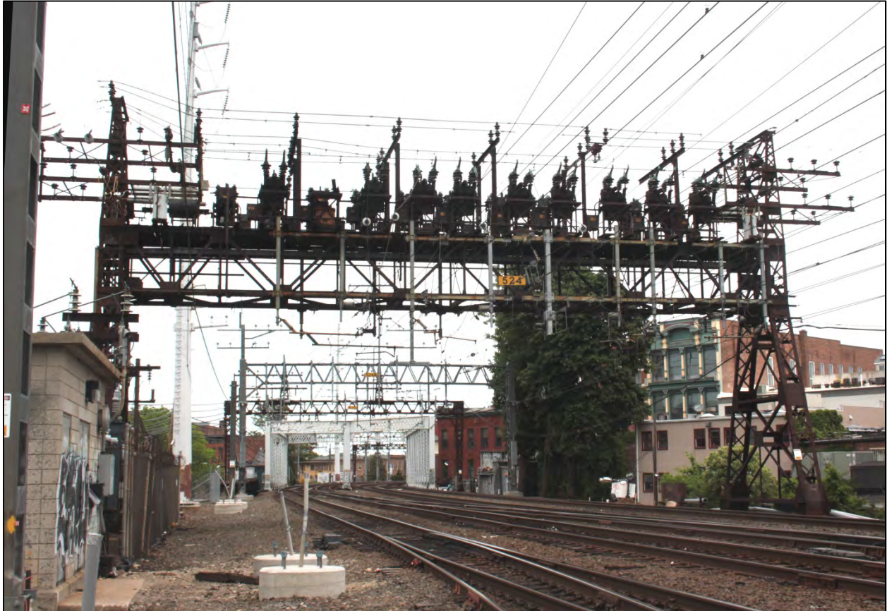
Photograph 1: Anchor bridge (sectionalizing bridge), Bridge 524, overview, camera facing northeast.
