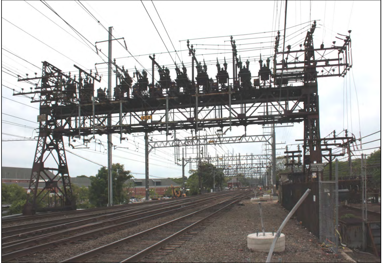
Photograph 2: Anchor bridge (sectionalizing bridge), Bridge 524, overview, camera facing southwest.
