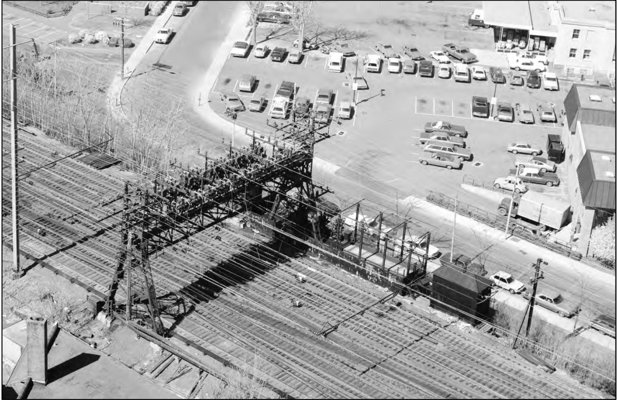
Figure 11: Anchor Bridge 524 (sectionalizing bridge) looking northwest, 1977, Historic American Engineering Record photograph by Jack E. Boucher, “Northeast Railroad Corridor, Amtrak Route between New York/Connecticut & Connecticut/Rhode Island State Lines” (HAER No. CT-11).
