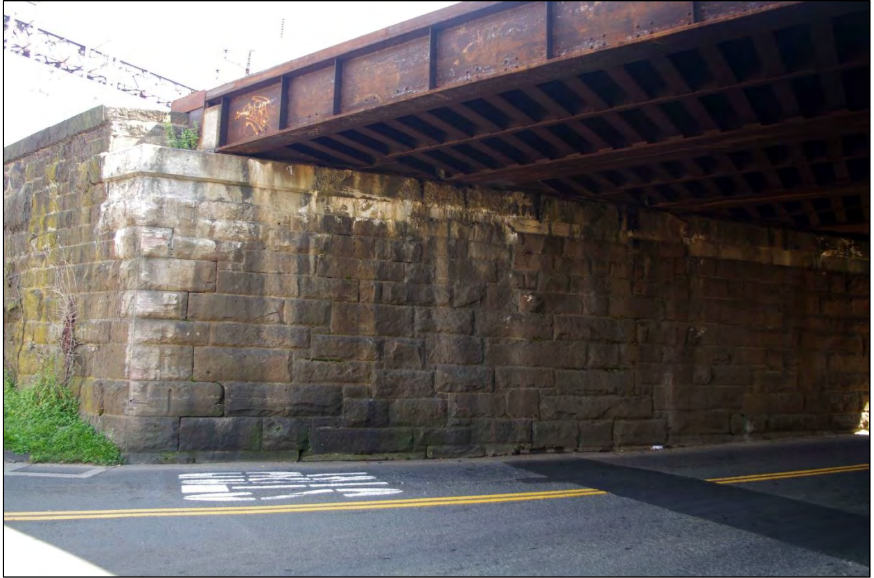
Figure 6. Fort Point Street Railroad Bridge, east abutment with ashlar stone masonry, camera facing southeast (AHS photograph, 9/2017).
