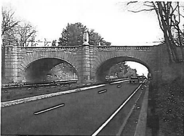
James Farm Road Bridge
